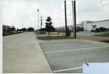
Pervious concrete at EBR Professional Development Center, Baton Rouge, LA
